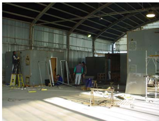
Modules prefabrication
