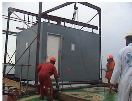
Modules installation on board
